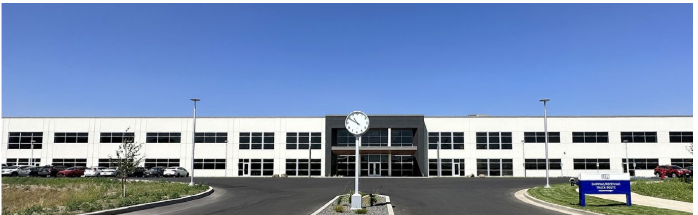
Schweitzer Engineering Laboratories' 162K-square-foot, $100M manufacturing facility in Moscow, Idaho.
