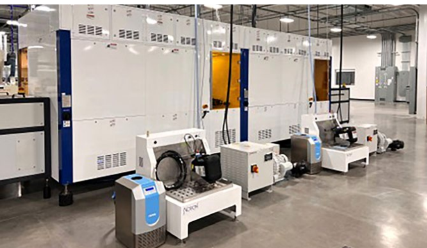
Figure 4: The machine set up at Schweitzer Engineering Laboratories' new facility in Idaho. (Source: SEL)
